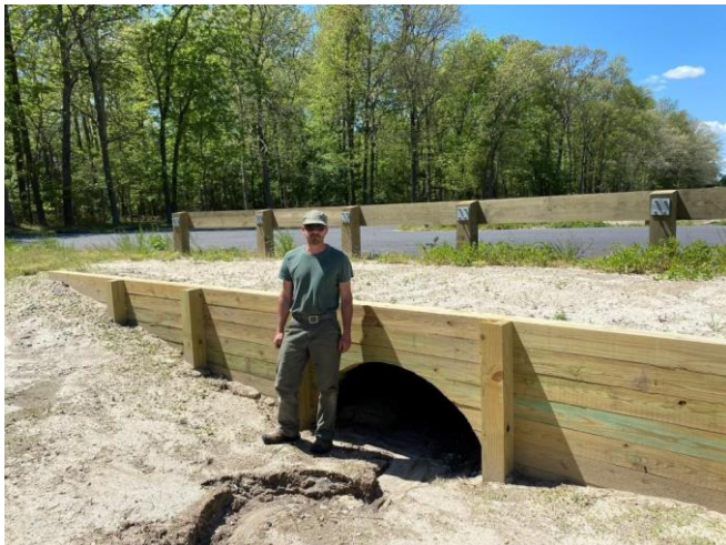
Jeremy Cole at the new culvert
